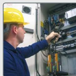
Almost every current asset which is supported by energy turns hot before a breakdown. Temperature monitoring can best be provided in line with preventive electrical maintenance.
